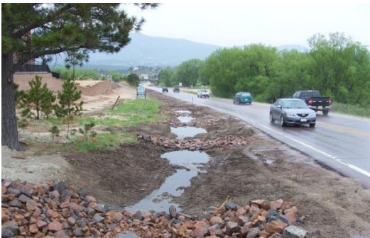
Excellent installation of rock Check Dams.
